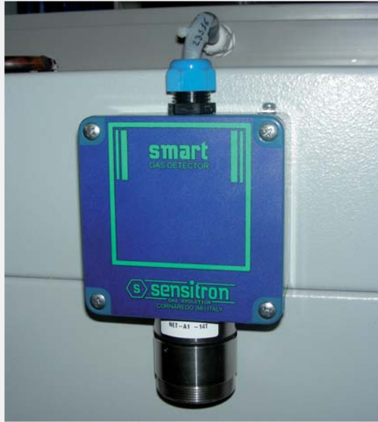
Dangerous gas (H 2 ; O 2 ; CO; CO 2 ;...) sensors
